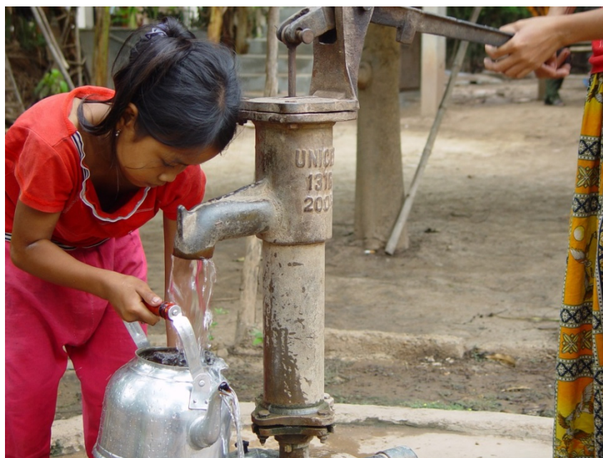
Shallow drinking water tube well in the Red River Delta, Vietnam, a region that is affected by naturally occurring (geogenic) arsenic contamination of groundwater
